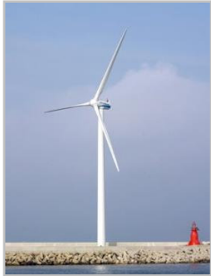
· 1.65MW wind turbine in the Ulsan shipyard
